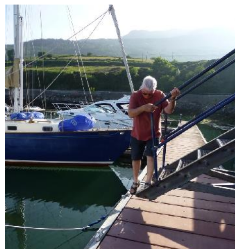
Carlingford Marina access stairs. They actually ended up over the water!
